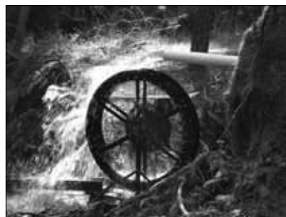
Micro-hydro system, a renewable energy system.
